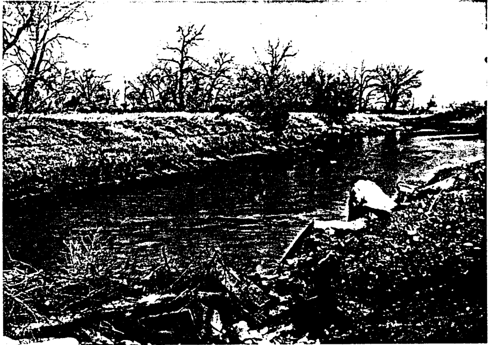
Milk River 1/4 Mile Downstream From Treatment Plant (remnants of washed out weir in foreground).
