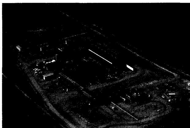
The Yellow Jacket central facility processes 210 million cubic feet of CO 2 per day prior to delivery to the Cortez Pipeline.
