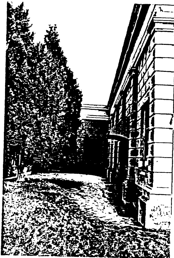
Figure 10: Looking east at north wall of main structure.
