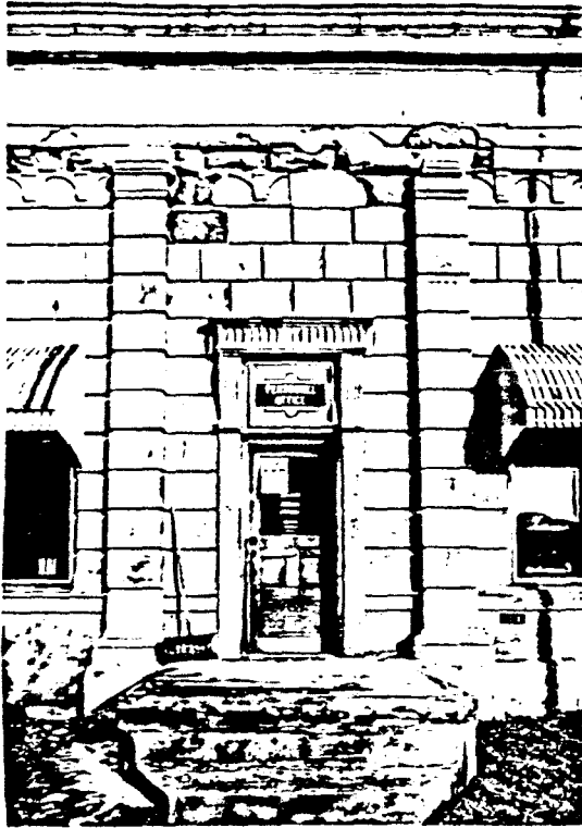
Figure 5: Spalled area over personnel office entrance on the west side.
