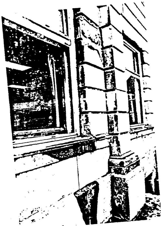
Figure 11: Looking at detail of spalled area on north side.
