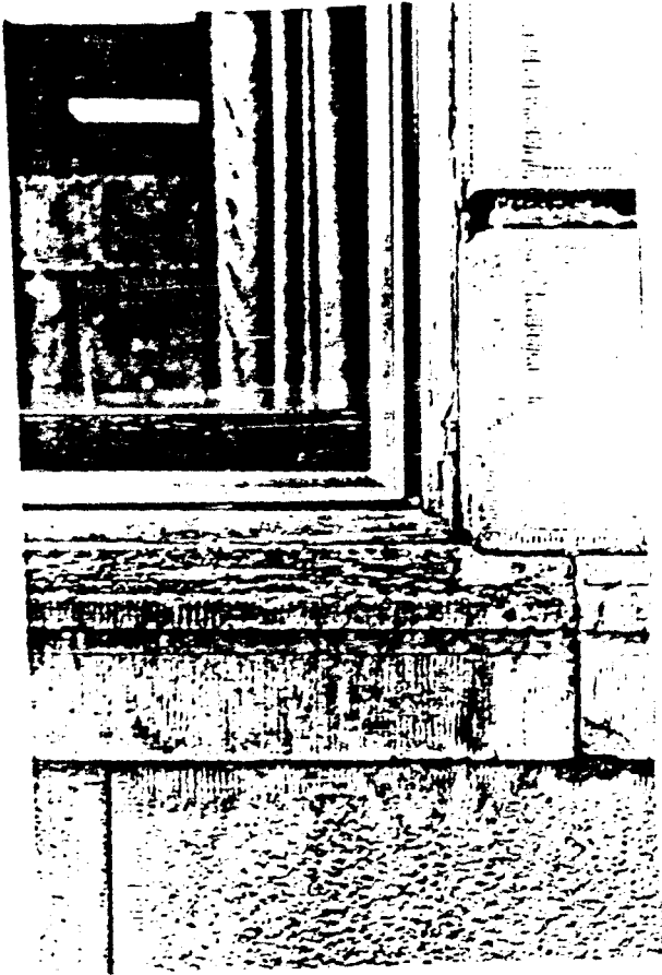
Figure 13: Detail of sill under window. Discoloration of surface denotes water penetration from water above.
