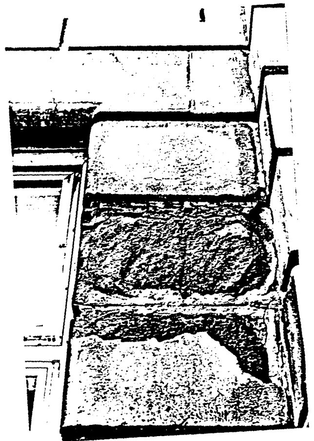
Figure 12: Detail of spalled surface on north wall.
