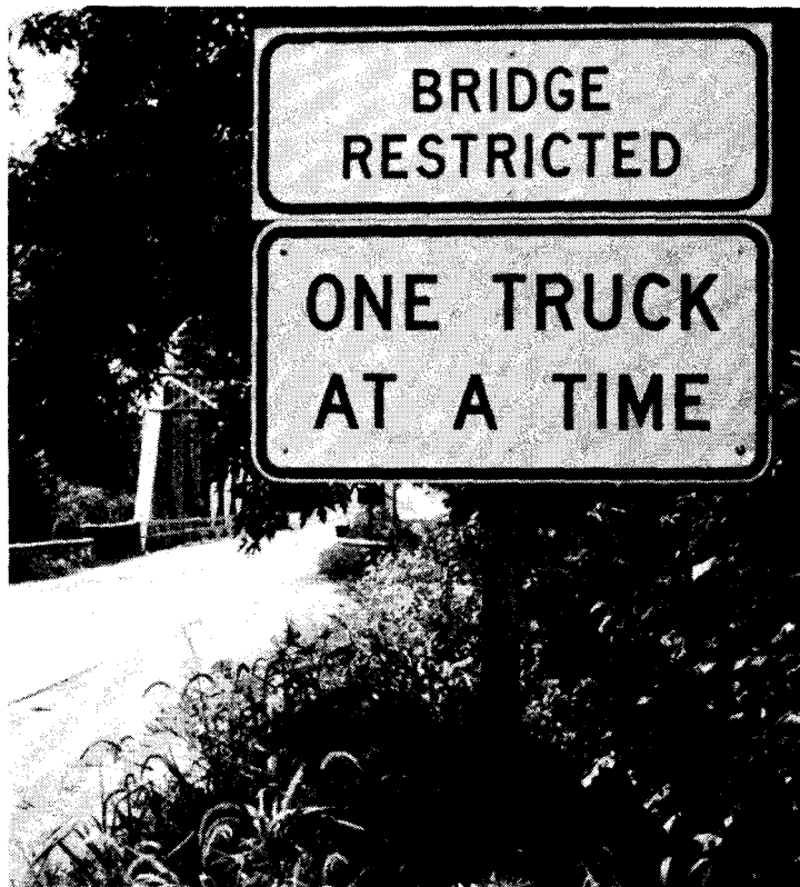
Only eight percent of the highway bridges in the nation are strong enough to handle 80,000 pound trucks without a decrease in service life.
