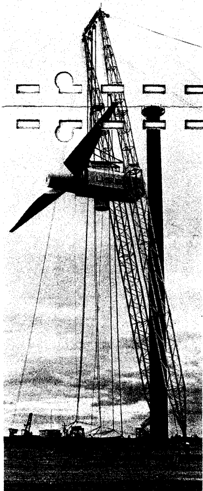
Hoisting of wind turbine
