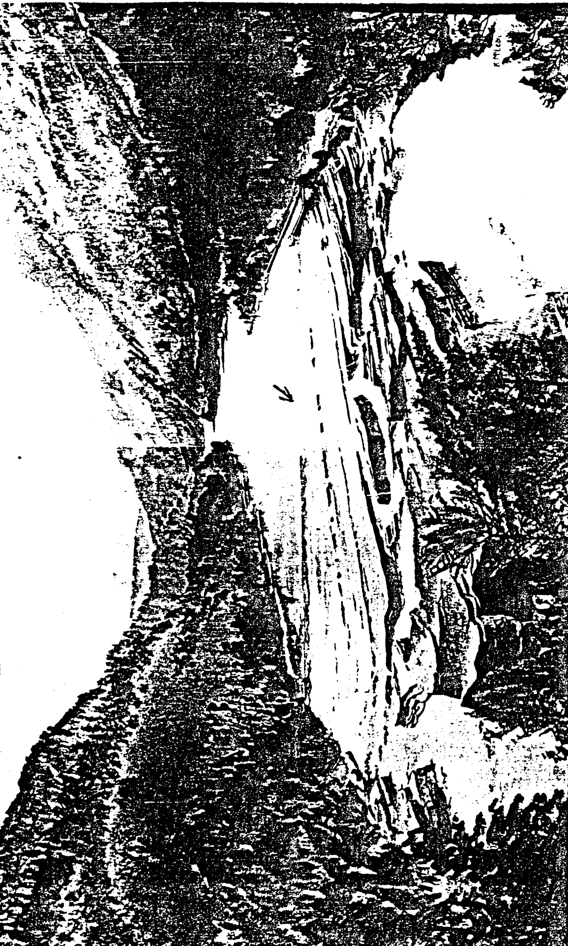
ARTIST'S CONCEPTION OF NORTHERN LIGHTS PROPOSED RUN-OF-THE-RIVER KOOTENAI RIVER HYDRO-ELECTRIC PROJECT IN OPERATION SHOWING UNDERWATER SPILLWAY. (SEE ARROW ON PICTURE) POWERHOUSE WILL BE UNDERGROUND.
