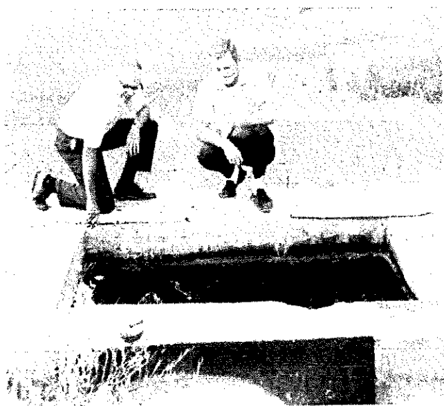
→ Figure 9.—Outlet for Town and Marks artesian well, flowing 3,700 gpm from the Tensleep. (Bob Marsh, Gary Knudson, left to right.) In the background are fields irrigated with water from this well.
