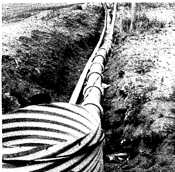
→ Figure 10.—Diversion pipe, Town and Marks well.
