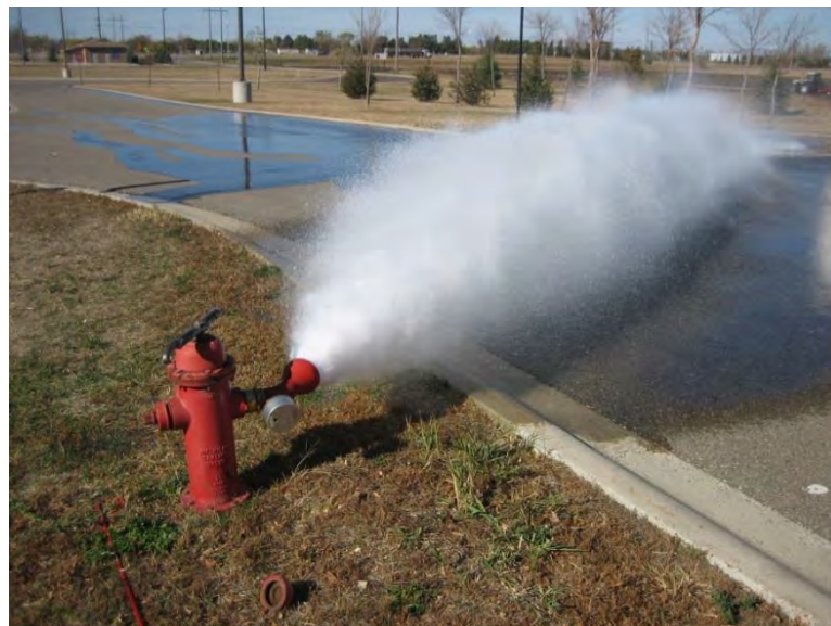
Figure 4-5: Operation of a Flowed Hydrant
